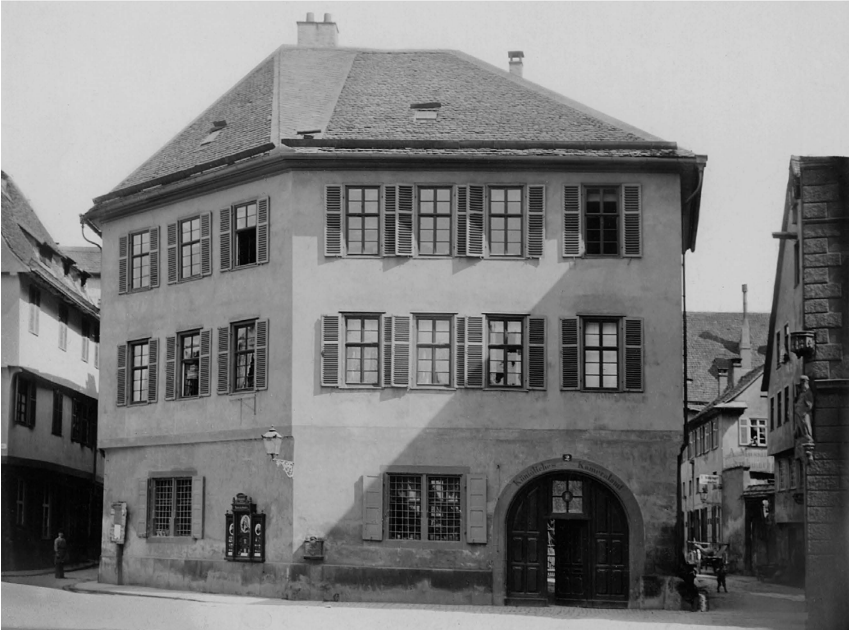
Old Cameral Office, prior to demolition, 1894
