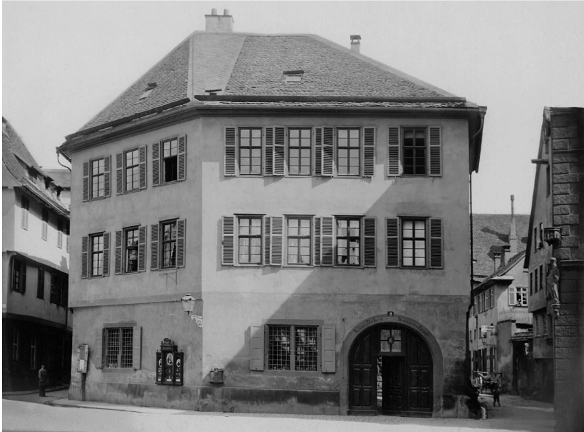
Old Cameral Office, prior to demolition, 1894
